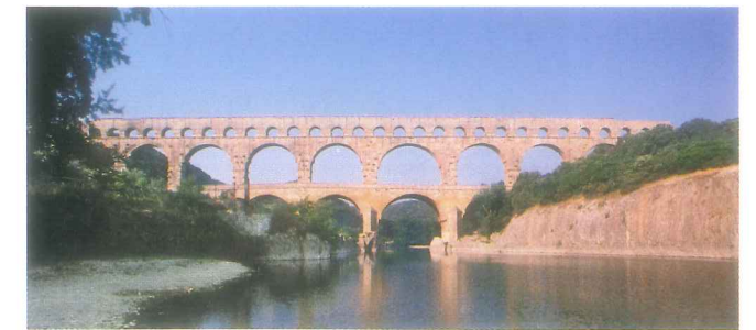
ROMAN AQUEDUCT IN SOUTHERN GAUL (FRANCE). Aqueducts conveyed water from mountains and lakes to the larger cities of the Roman Empire. The massive arches shown here were originally part of a 31-mile-long complex that supplied water to the city of Nemausus (Nîmes). It is now known as the Pont du Gard (Bridge of the Gardon), reflecting the use to which it was put after the aqueduct ceased to function, some eight centuries after its construction in the first century C.E. Many Roman aqueducts remained operational into the modern era: the one at Segovia, Spain was still in use at the end of the twentieth century. ■ What does the magnitude and longevity of such projects tell us about Roman power and technology?
